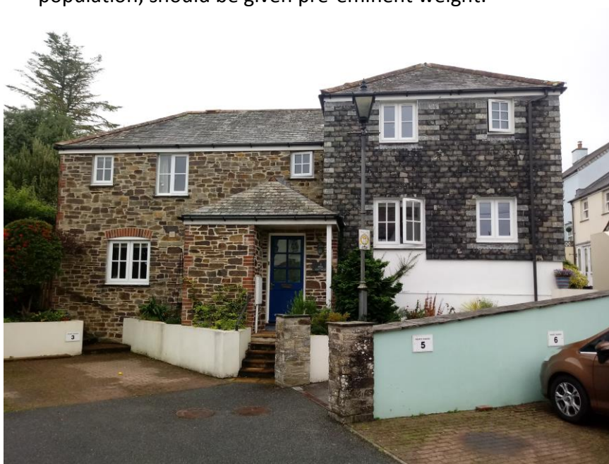
The award-winning Lemon Hill Gardens development which responded to the neighbouring properties by incorporating a range of Cornish architectural references
